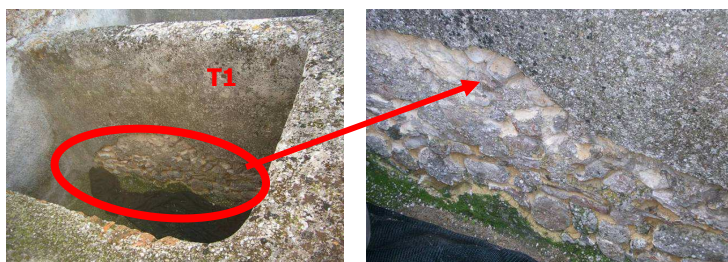
Figure 2 – Application of T1 mortar in the Cetariae in the inland area
