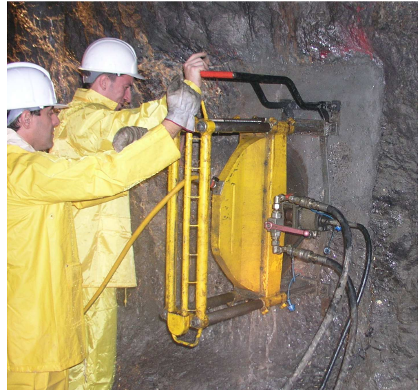
Fig. 7 – SFJ slot cutting device with the oil engine
