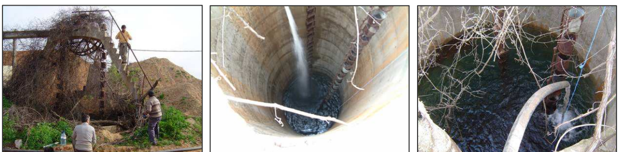
Figure 4 – Injection test developed in the “nora”: water levels at the beginning and at the end of the test
