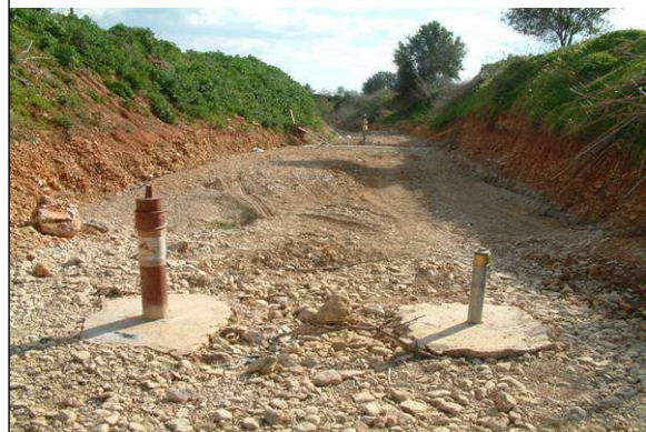
Figure 7 - Design configuration of the two infiltration basins in the river bed of rio Seco (Carreiros)
