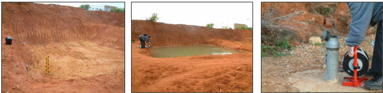
Figure 3 – Infiltration basin in the second layer and monitoring equipment used for the infiltration test
