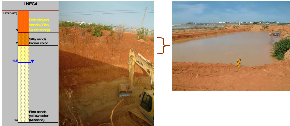
Figure 2 –Vertical profile of lithological materials in Areal Gordo (at right) and LNEC4 well lithological column and, infiltration basin in the first layer (at left)
