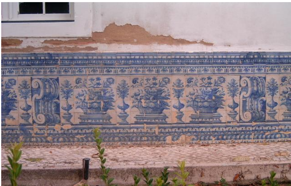
Figure 2- Salt crystallization above a street azulejo panel at Casa dos Patudos (photo by Manuel Anastácio, Wikimedia)
