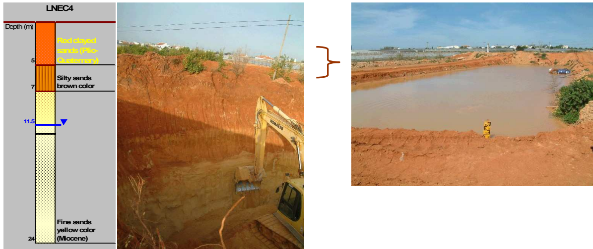
Fig. 2 –Vertical profile of lithological materials in Areal Gordo (at right) and LNEC4 well lithological column and, infiltration basin in the first layer (at left)
