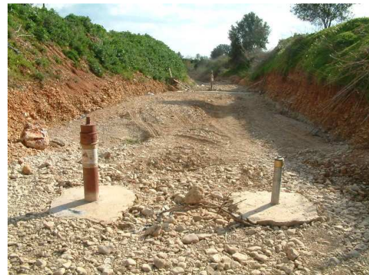
Fig. 14 - Design configuration of the two infiltration basins in the river bed of rio Seco (Carreiros)
