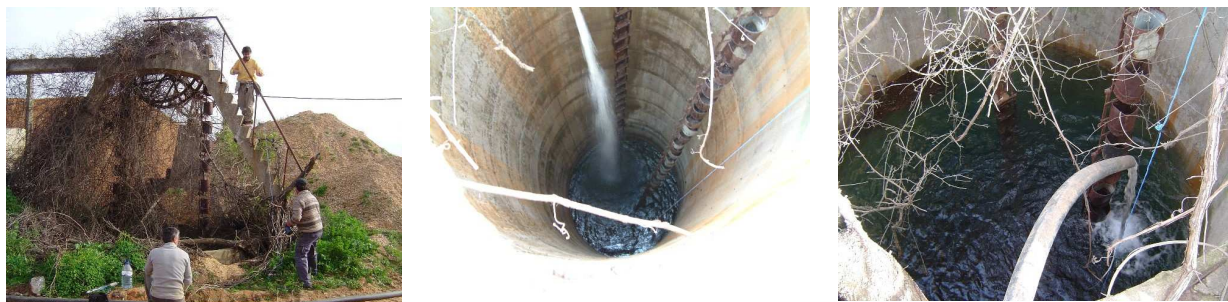
Fig. 10 – Injection test developed in the “nora”: water levels at the beginning and at the end of the test
