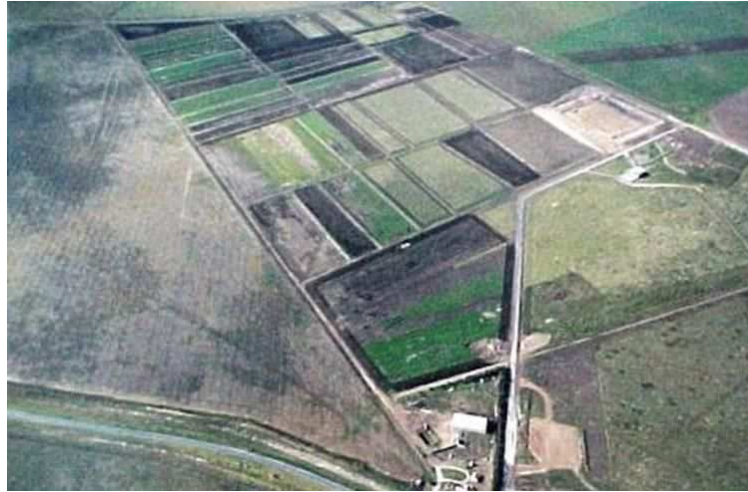
Fig. 42 - IPES Industrial waste treatment plant
