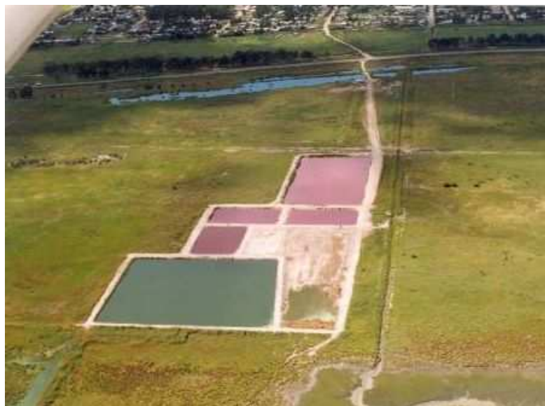
Fig. 41 - Siracusa slaughterhouse's water treatment plant
