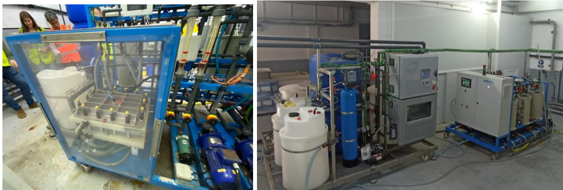
Figure 4: Right: Selective electrodialysis membrane stack; Left: Brine valorisation pilot plant installed at Rincón de León WWTP.
