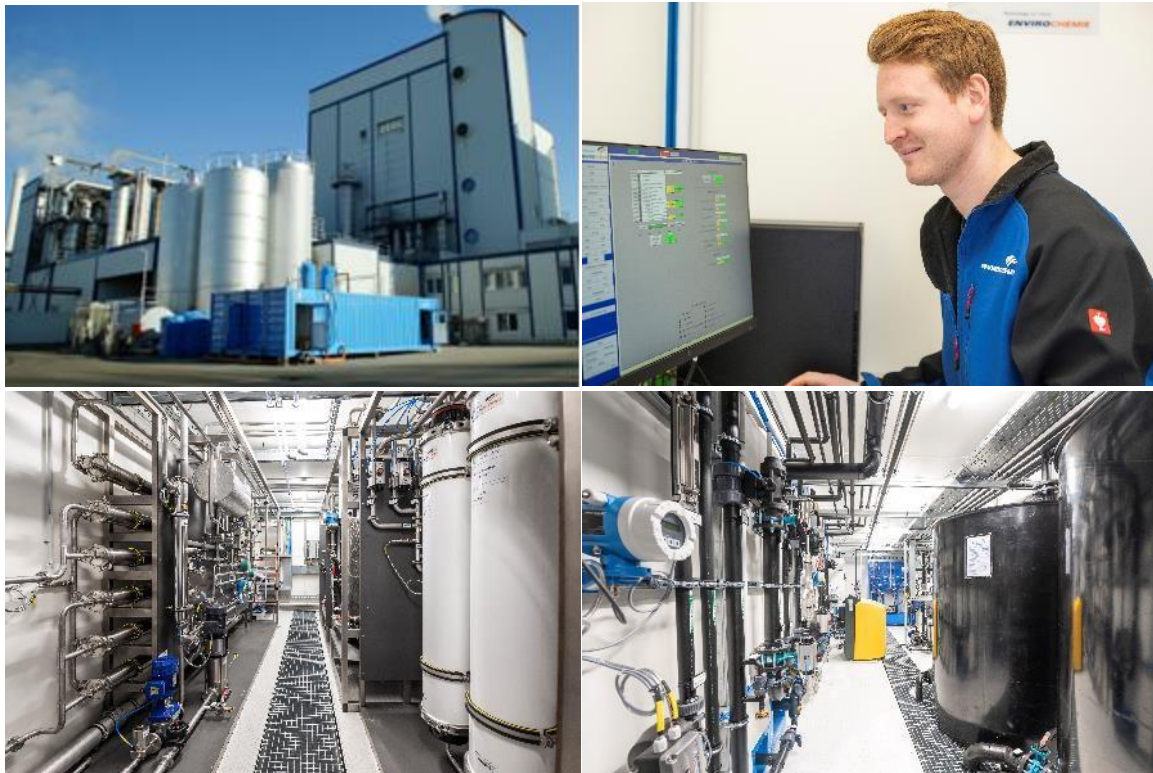
Figure 12: Impressions of the pilot plant of LL East Frisia. The treatment technologies were located in the blue containers. The inside of the containers is depicted below.
