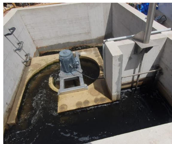
Figure 3: Left: Conceptual design of spiral basin and turbine. Right: final setup of the picoturbine installed at Monte Orgegia WWTP.
