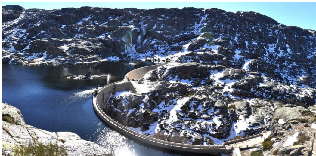
Figure 3.1: Covão do Meio dam. View from the right bank in winter
