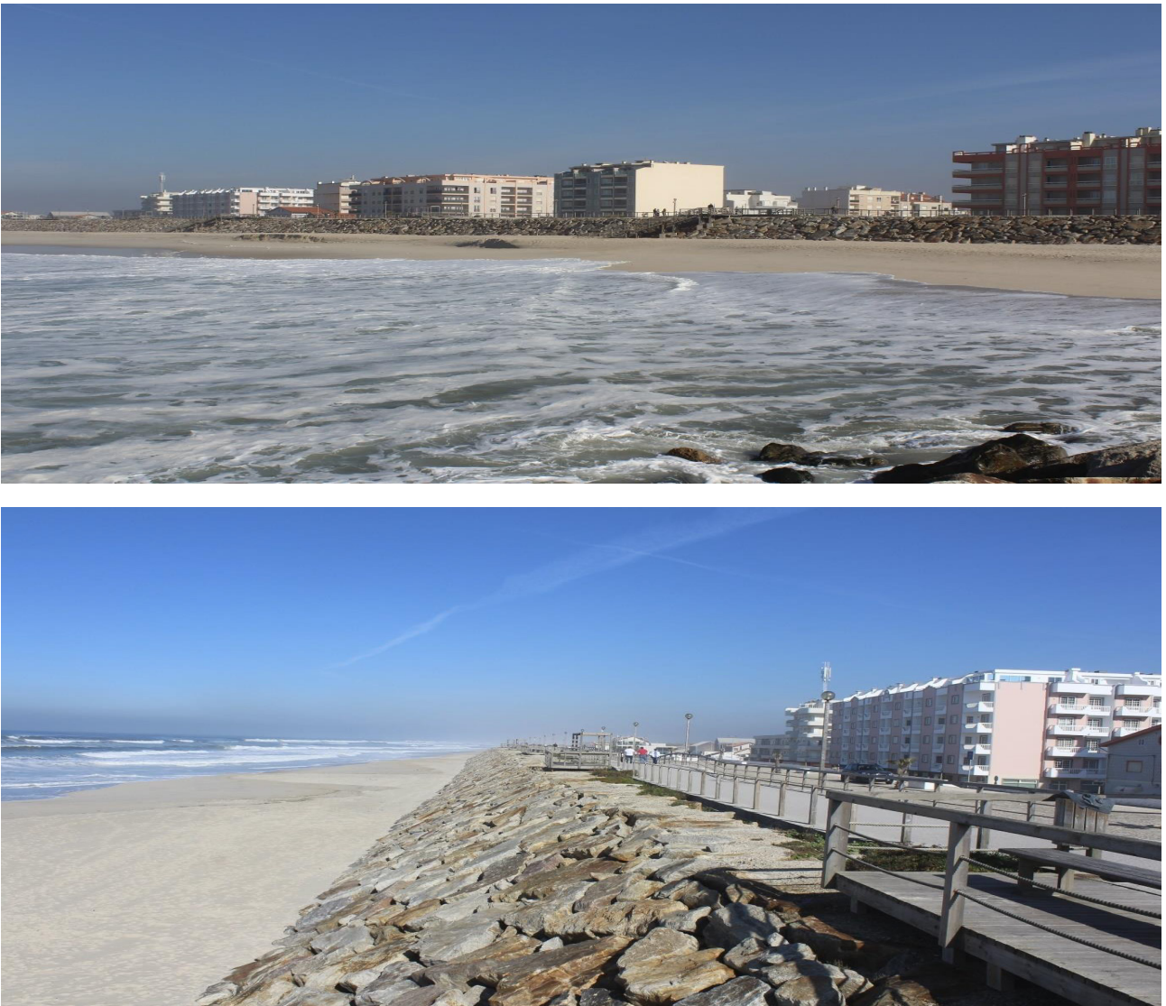
Figure 1. View of the longitudinal frontal defence structure of Vagueira beach (Rosa, 2021).
