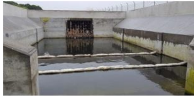
Intervention finished in February 2021
