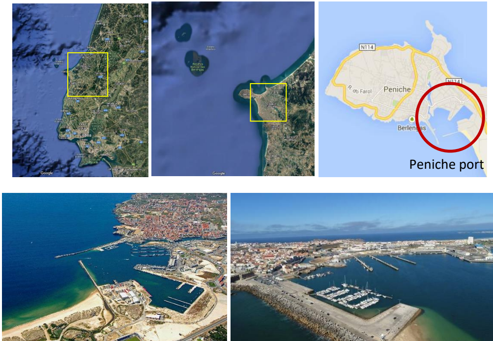
Figure 3 – Port of Peniche. Location and aerial views of the port.
