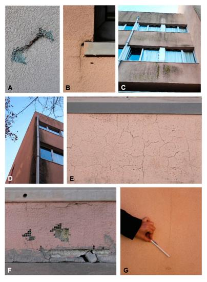
**Figure 3.** Relevant anomalies identified on the façades: (A)—perforation of the system; (B)—cracking of the rendering system in window openings; (C)—biological colonization; (D)—water runoff marks; (E)—non-oriented cracking; (F)—detachment of the finishing coat; (G)—oriented cracking.
