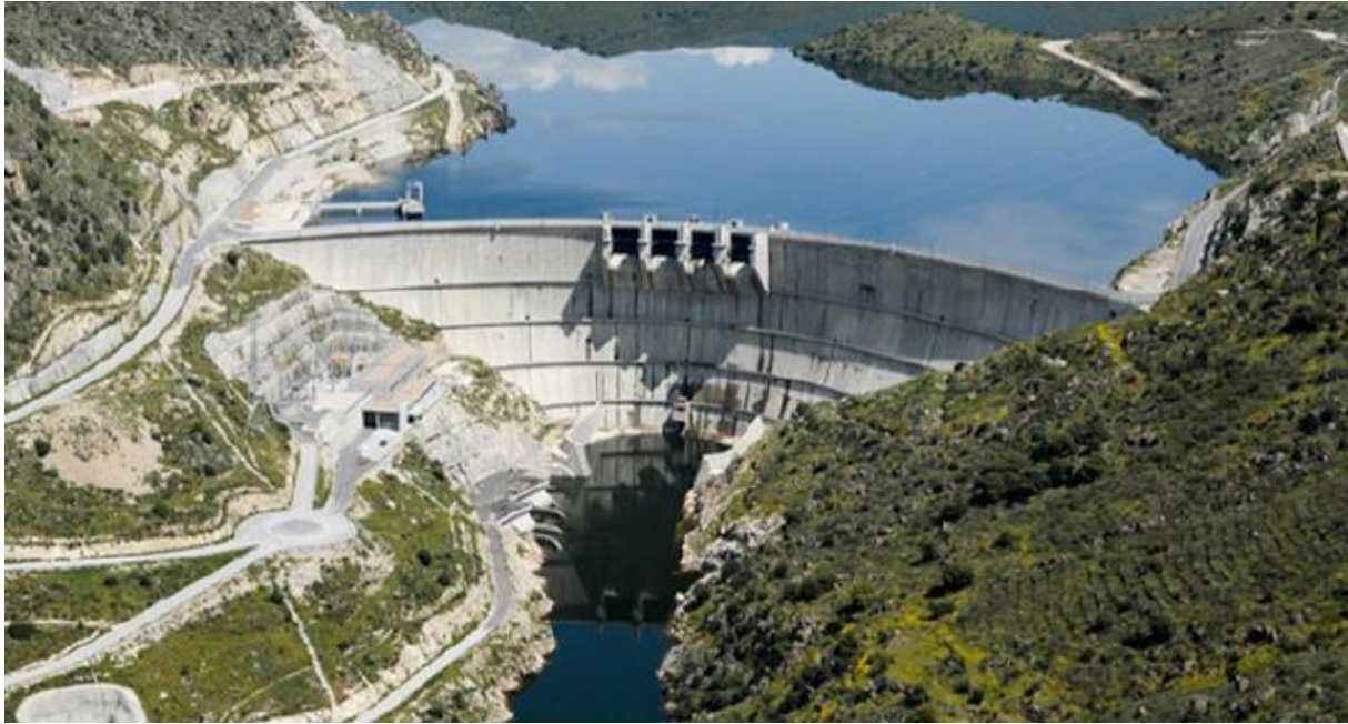
Figure 74 – Baixo Sabor concrete arch dam (LNEC, 2017b).
