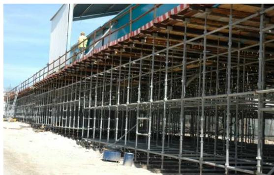
**Fig. 1:** Example of bridge falsework Cuplok® systems
