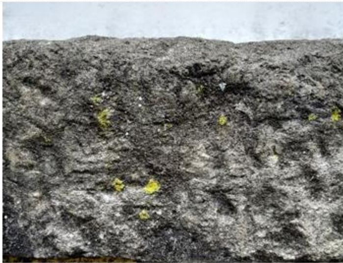
Figure 18: Colonization of the stone by lichens. Source: authors' file, 2021
