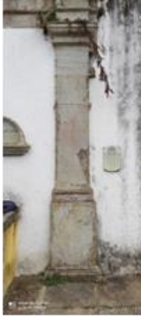
Figure 6: Both pictures from the column on the left side of the fountain, with the highest concentration of degradations. Source: authors' file, 2021.
