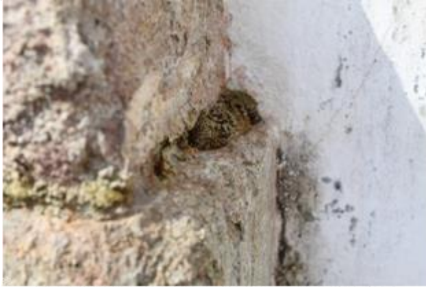
Figure 20: Colonization of moss at the column joint: authors' file, 2021.
