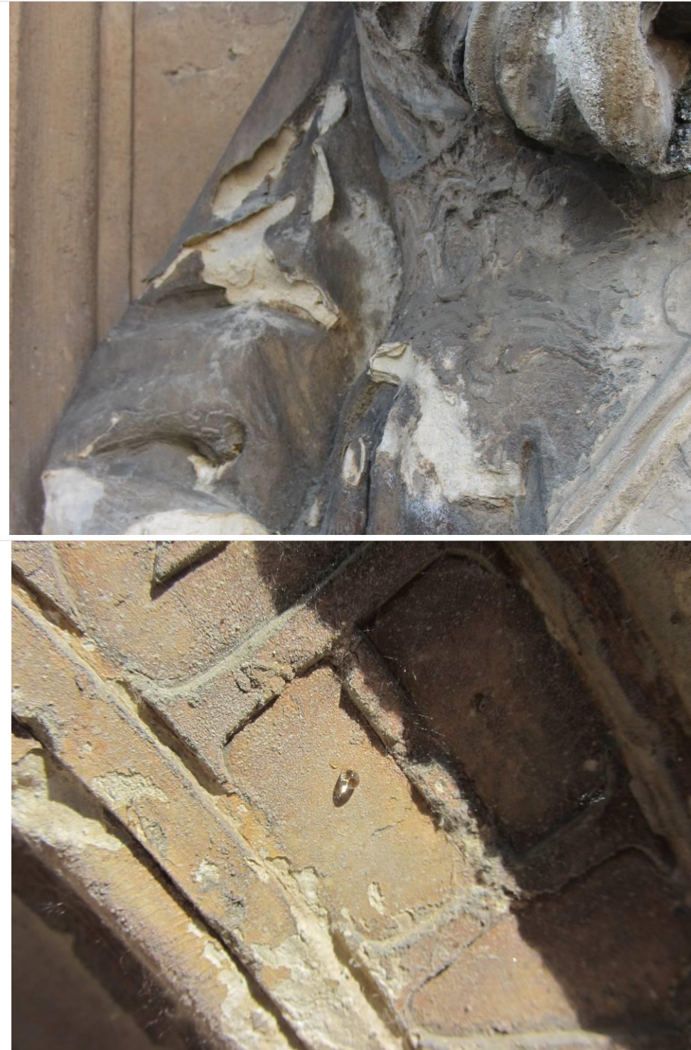
Figure 3 – Sound surfaces should not be consolidated as strength reinforcement is not logically justified, its presence is not innocuous and can compromise the long-term performance due to excessive incompatibility
