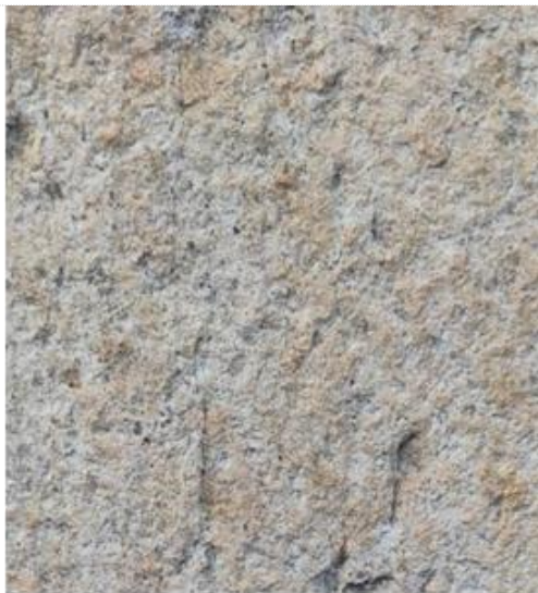
Figure 4: Detail of texture, color and granulometry of Itacolomy quartzite at Chafariz da Glória . Source: authors' file, 2020.
