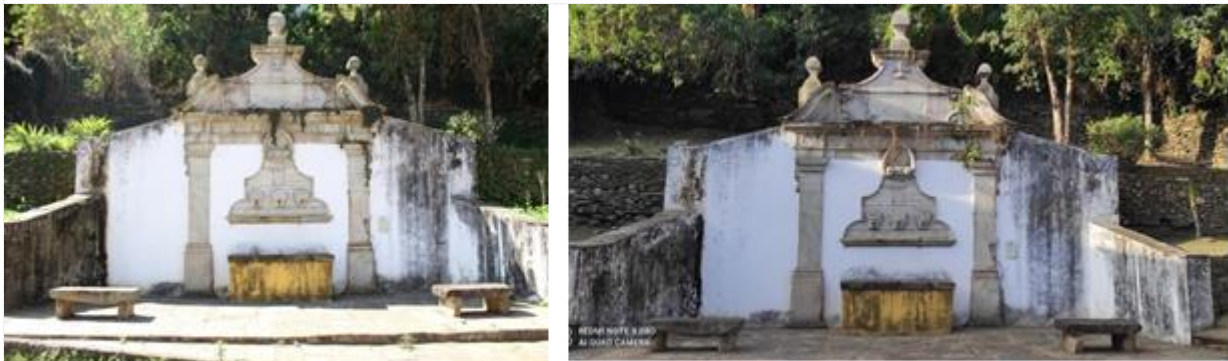
Figure 2: Incidence of solar radiation at Chafariz da Glória at noon in July (left) and in the afternoon at 4 pm (right). Source: authors' file, 2020
