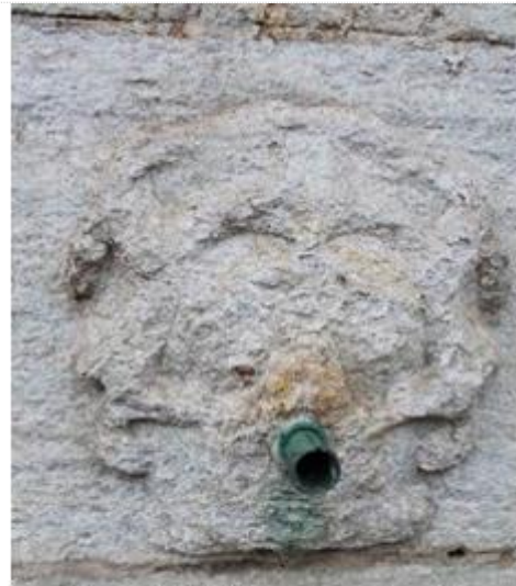
Figure 15: Scaling and erosion, with rounding of vertices and edges. Source: authors' file, 2021.
