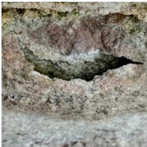
Figure 16: Blistering (stuffing). Source: authors' file, 2021.
