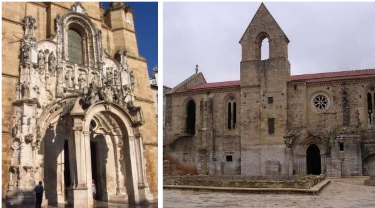
Fig. 1 – Aspect of “Ançã stone” in the Renaissance portal of Santa Cruz church, Coimbra (left), and of “Coimbra dolostone” in the Santa Clara old convent, Coimbra (right).
