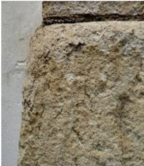
Figure 14: Quartzite swelling and breakdown. Source: authors' file, 2021.
