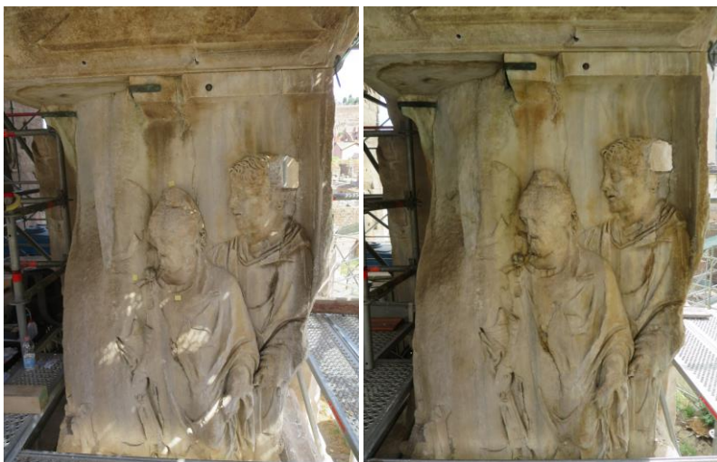
Fig. 1: West plane of the plinth before (left) and after (right) the biomineralisation treatment.
