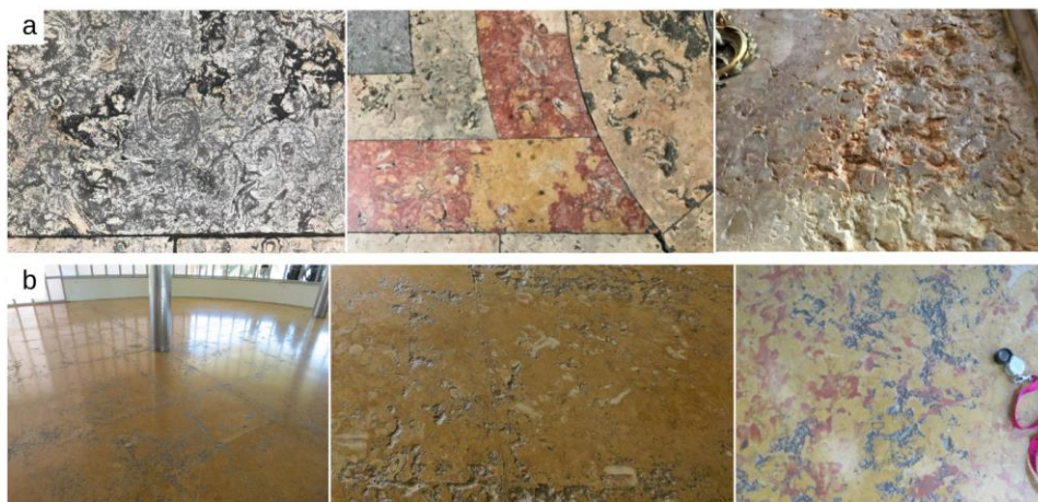
Figure 04: Photographs of internal floor and wall covering (right) applications of the Lioz inside the Basilica da Estrela , in Lisbon, Portugal (a), and of the internal floor of the Museum of Modern Art, in Belo Horizonte, Brazil (b). The rocks present chromatic variations, presence of fossils, differential erosion and loss of matrix (Photo: Antônio Gilberto Costa).
