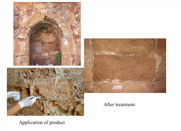
Fig.1_ Consolidation treatment with TEOS-CaOx.
