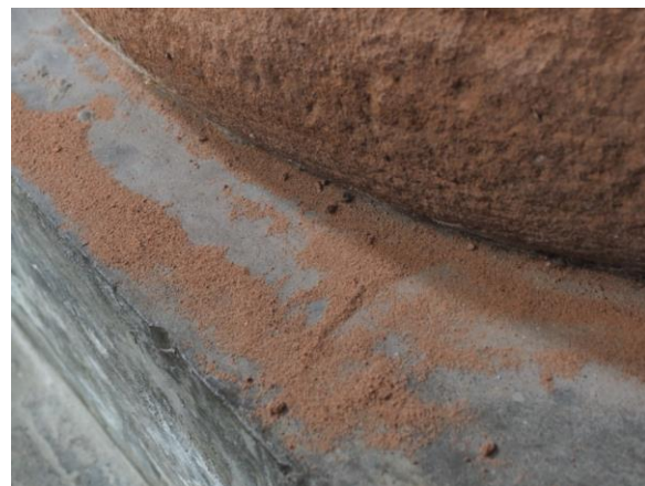
Fig. 3 Sanding of stone (sandstone), photo from MDCS
