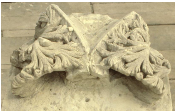
Figure 12. Burrell Collection French doorway (Reg. No. 44/89). Fragile stonework block photographed in 1981, prior to consolidation (photo: Deborah Carthy).
