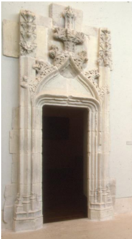
Figure 11. Burrell Collection French doorway (Reg. No. 44/89). Darkening of the stone in the upper central fragile area after consolidation (photo: Glasgow Museums).
