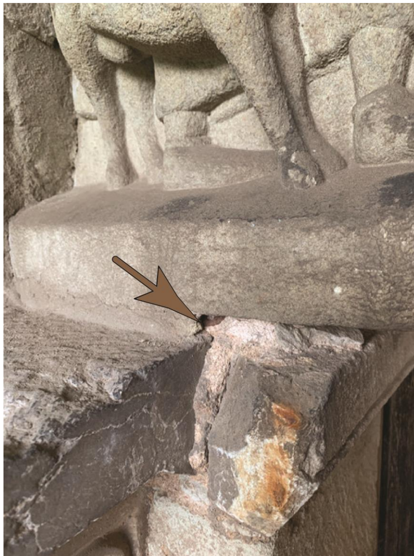
Figure 5. Aston Eyre Church tympanum. Detail of the sand/silane mortar mix at the base of the sculpture. The arrow shows the cavity where the mortar powdered away when gently probed in 2020 (photo: Deborah Carthy).
