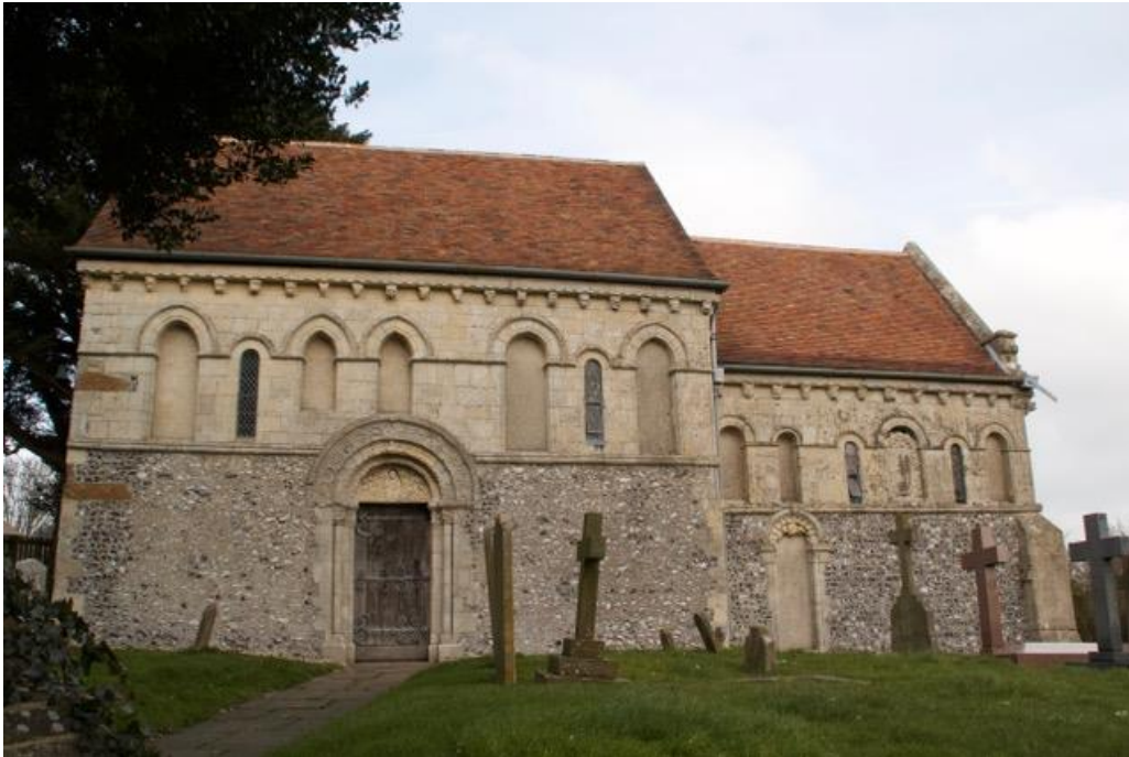
Figure 13. St Nicholas Church, Barfrestone. The south-facing aspect showing the consolidated doorway and the adjacent, unconsolidated minor doorway in 2019 (photo: Deborah Carthy).
