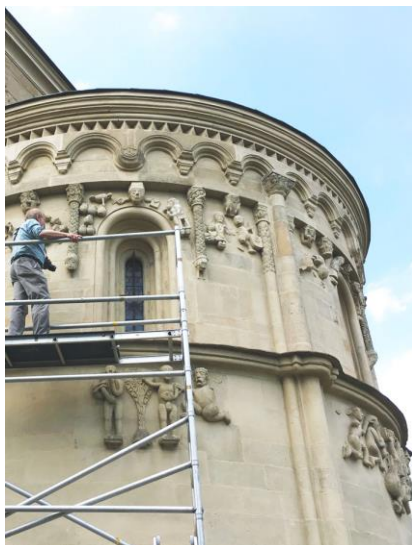
Figure 8: translucent sacrificial lime-sand layer, applied on the sandstone façade of the apse of the Romanesque church of Schöngrabern, Lower Austria, after completion of its conservation. The photograph was taken approx. 20 years later.
