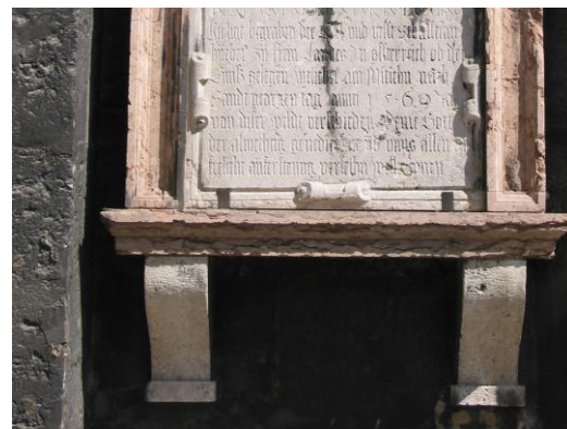
Figure 5: detail of an epitaph on the exterior façade of Vienna Cathedral; the photo, taken before conservation, shows four lithotypes of limestone with differing susceptibility to atmospheric impact. The red framing (Adnet limestone, regular variety with clayey veins) reveals the worst state of weathering.
