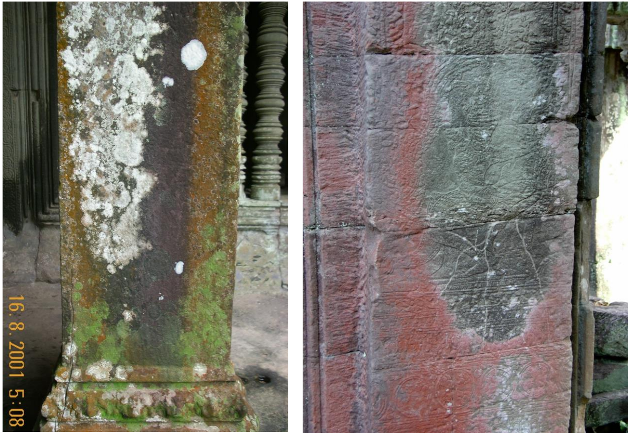
Figure 7 a + b: Natural multicolored biofilms of different photosynthetic microorganisms (e.g. lichens, algae and cyanobacteria) on Angkor monuments distinctly separated due to expositional factors and interspecific competition.
