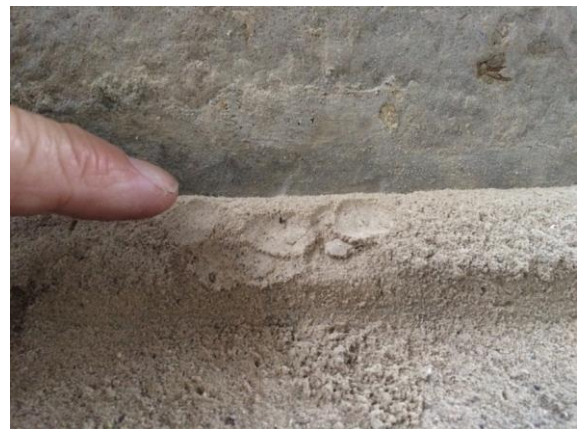
Fig. 2 Powdering of lime stone, photo from MDCS
