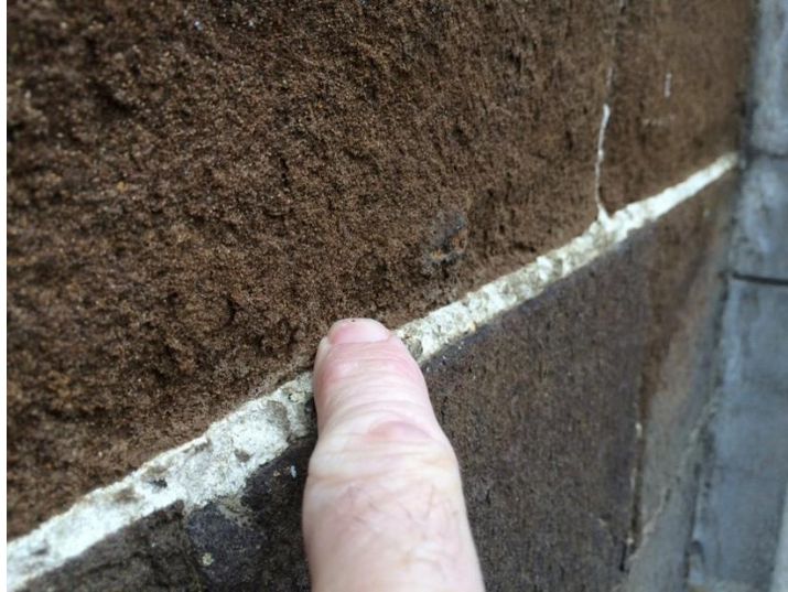
Fig. 5 In between stage of sanding and crumbling (ferruginous sandstone); photo from MDCS
