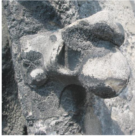
Figure 2a (top): crab at Vienna Cathedral, biocalcarene; characteristic features of weathering with gypsum crust in sheltered areas and surface erosion at exposed surfaces.
