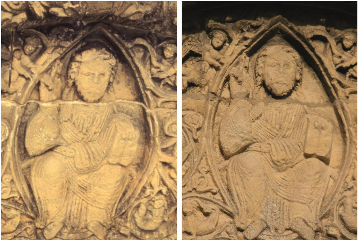
Figure 8. St Nicholas Church, Barfrestone. Detail of depiction of Christ in Glory at the doorway apex. Left; in 1977 after raking out the mortar but before consolidation, Right; in 2019 (photo: Left, Deborah Carthy; Right, Richard Cook).
