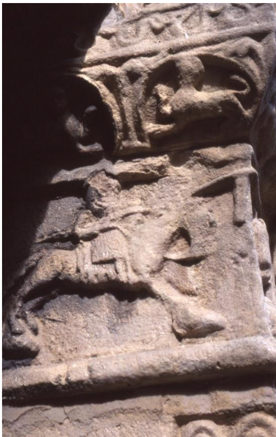
Figure 10. St Nicholas Church, Barfreestone. Detail of one of the many small carvings flanking Christ showing highlights in the photograph of 2004 where only very few small residues of silane were still visible on the surface (photo: Deborah Carthy).
