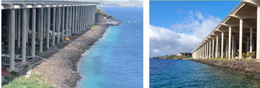
**Figure 1.** General view of the berm breakwater and the foundation columns of the airport runway extension, April 2021.
