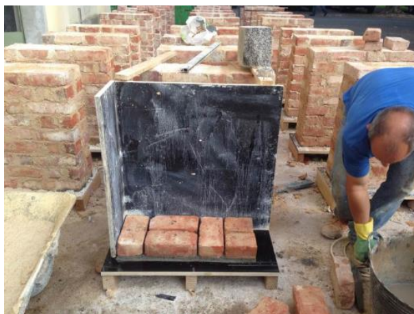
Figure 5. Execution of new solid brick wallettes.
