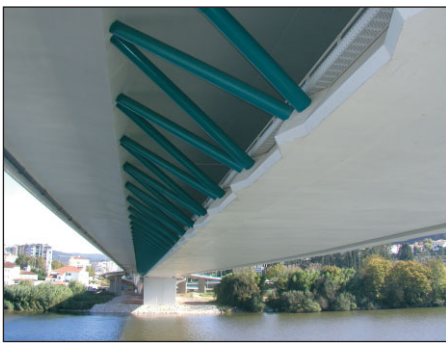
Fig. 3: View of the bridge deck cross-section
