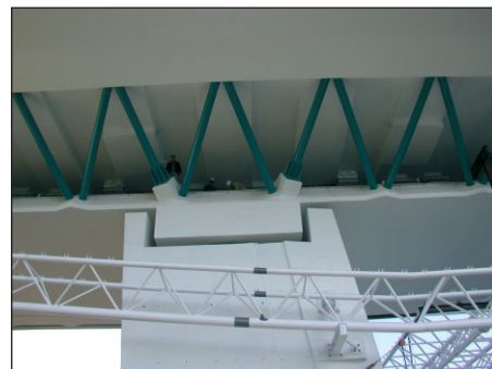
Fig. 2: Mast and deck support on pier P3
