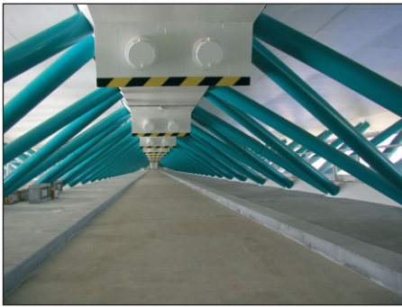
Fig. 4: The pedestrian walkway in the lower slab
