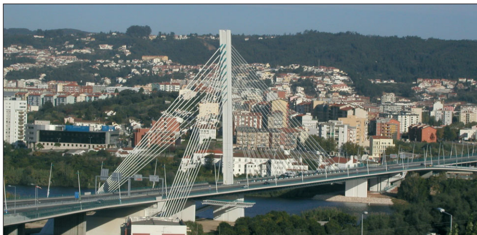
Fig. 1: General view of the bridge
