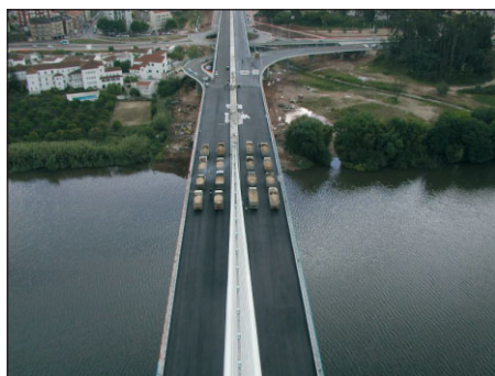
Fig. 8: Loaded trucks during tests
