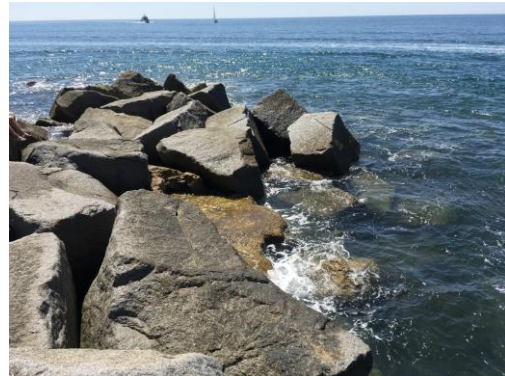
Figure 1 – Photograph taken during a visual observation campaign of a breakwater
