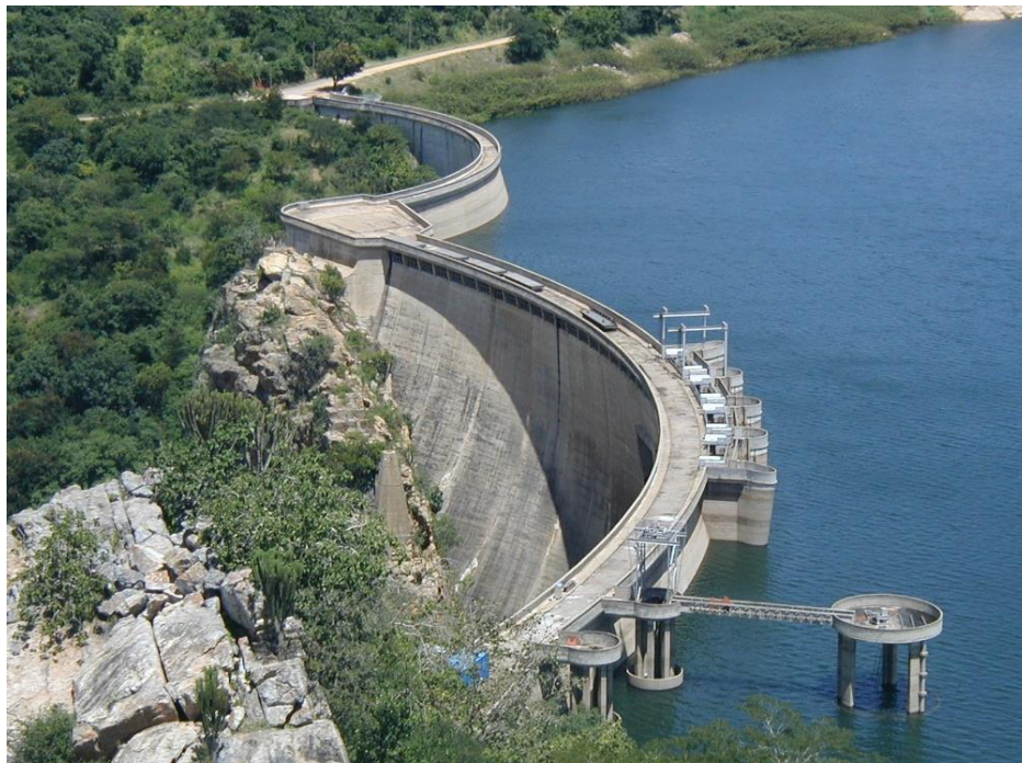
Fig. 1 – Chicamba dam. General view from the outcrop top at the left bank
