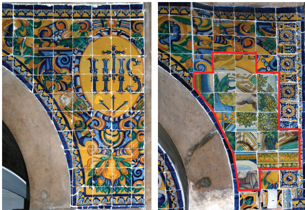
Figure 1. An arch spandrel orderly lined with Sevillian azulejos (left side) compared to another with intermixed azulejos (right side) – the tiles referred to in this paper are within the area outlined in red
