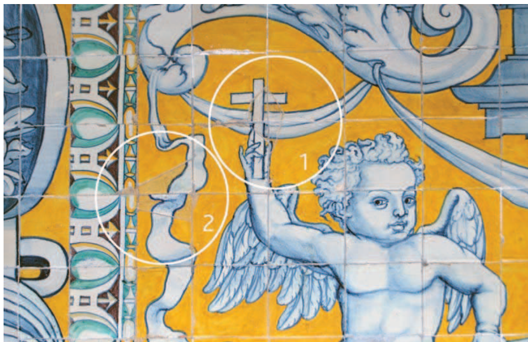
Figure 3. A detail of the panel of the putti showing two restored areas repairing a perforation (1) and evincing the different hue of the yellow pigment used (2)
