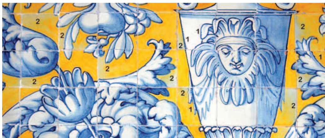
Figure 6. Evidence of technical issues in the panel of the dog: 1) running of the dark blue outlines; 2) blue or green staining
