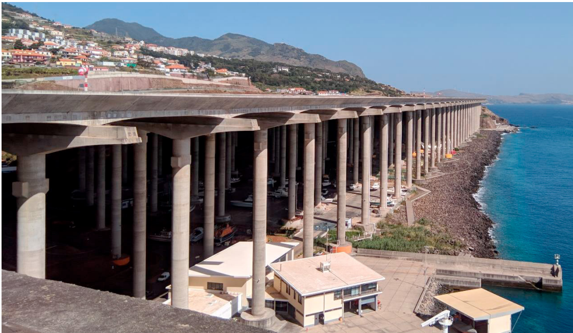
Fig. 1. Madeira Airport runway extension and its supporting structure.
