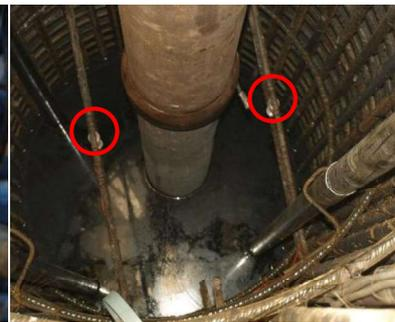
Figure 3.5: Strain gauges during concreting of a pile
