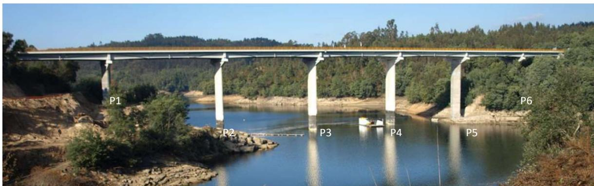
Figure 2.5: São João das Areias Bridge before the rehabilitation of the piers and foundations
