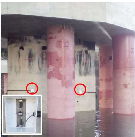
Figure 3.6: Strain gauges in an original pier
