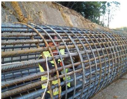
Figure 3.3: Rebar instrumentation at the construction site
