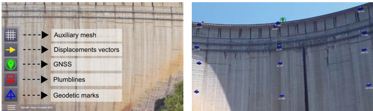
(a) Menu that allows the user to select which visual elements should be shown in the AR environment. (b) Network of sensors in the AR environment
