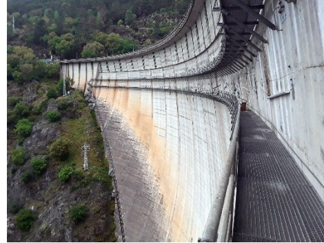
(b) Downstream face of the structure
