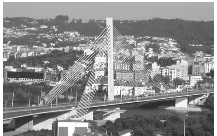
Figure 3. General view of the Coimbra cable-stayed bridge
