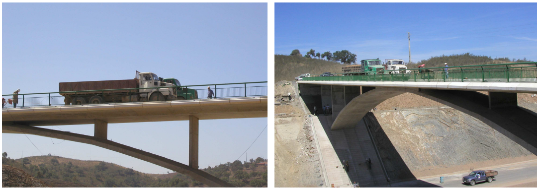
Figure 5 : Static load test
