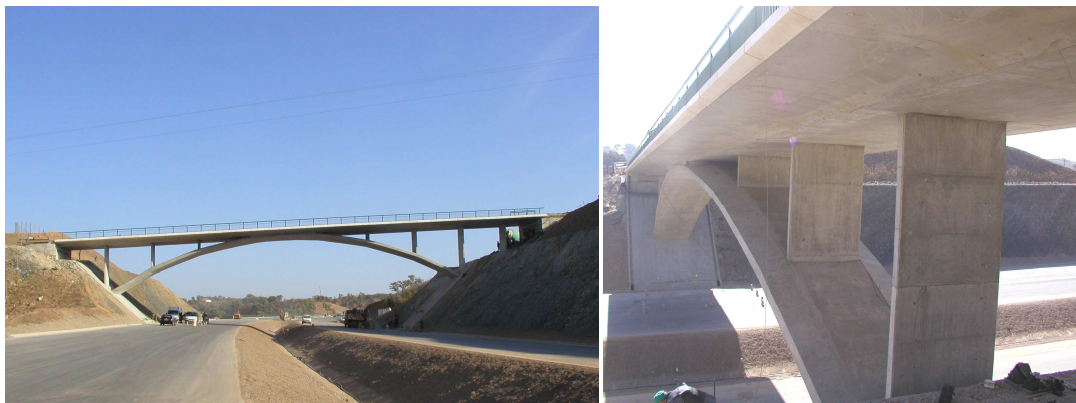
Figure 1 : The overpass bridge PS2
