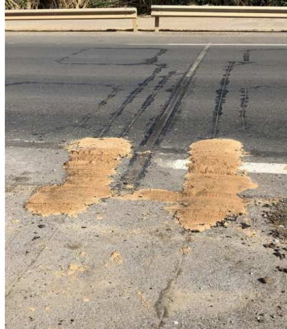
Figure 11. Devices installed in RN11 for weigh-in-motion testing (Macedo, A. et al. 2019)
