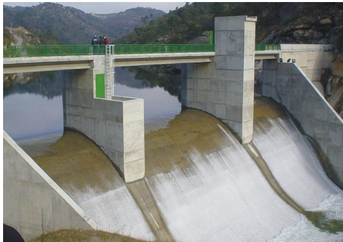
Figure 3: Downstream view of Bouçoais-Sonim dam
