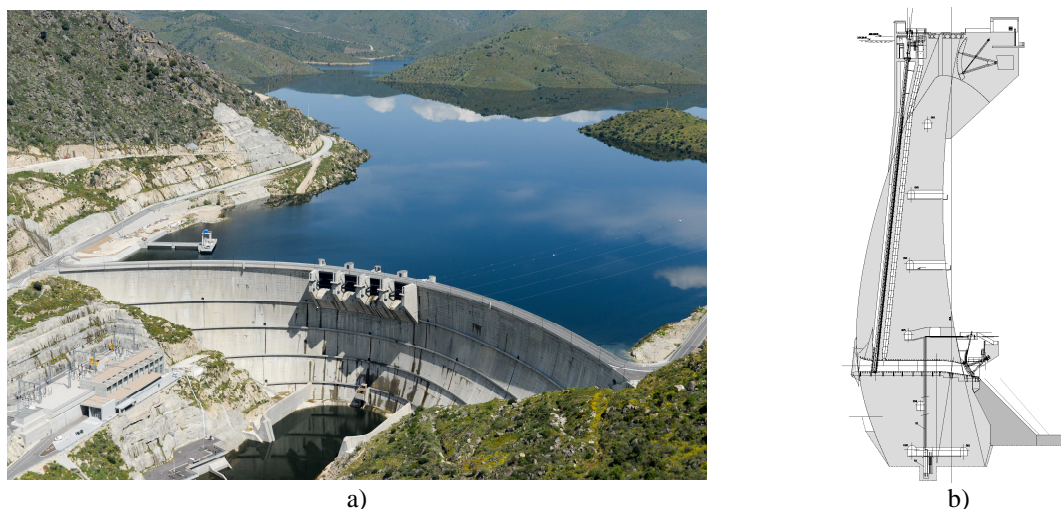
Figure 1: Baixo Sabor dam, a) aerial view after the first filling of the reservoir, b) cross section through the bottom outlet
