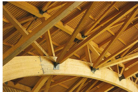
Fig. 3 Timber structure, including a section of an arch
