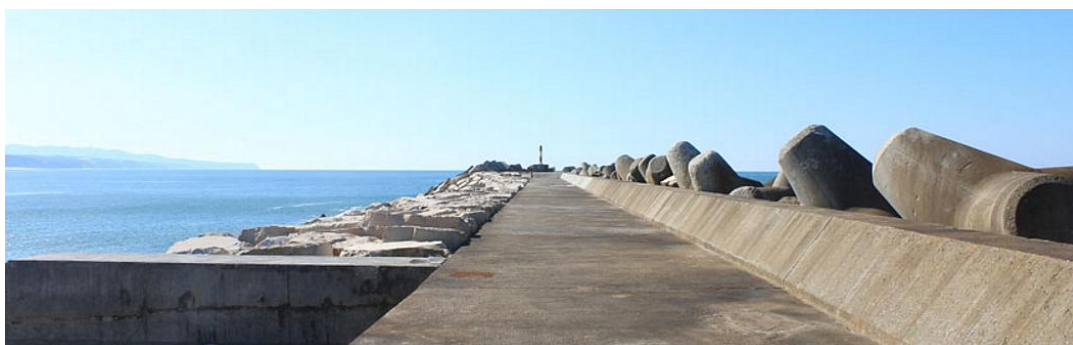
Fig. 2 Superstructure of Ericeira north breakwater
