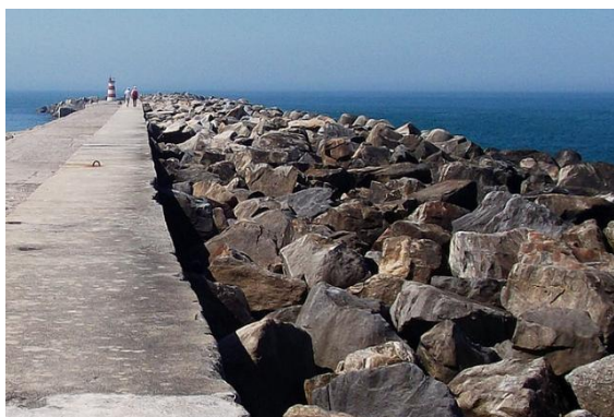
Fig. 3 Seen from the superstructure
