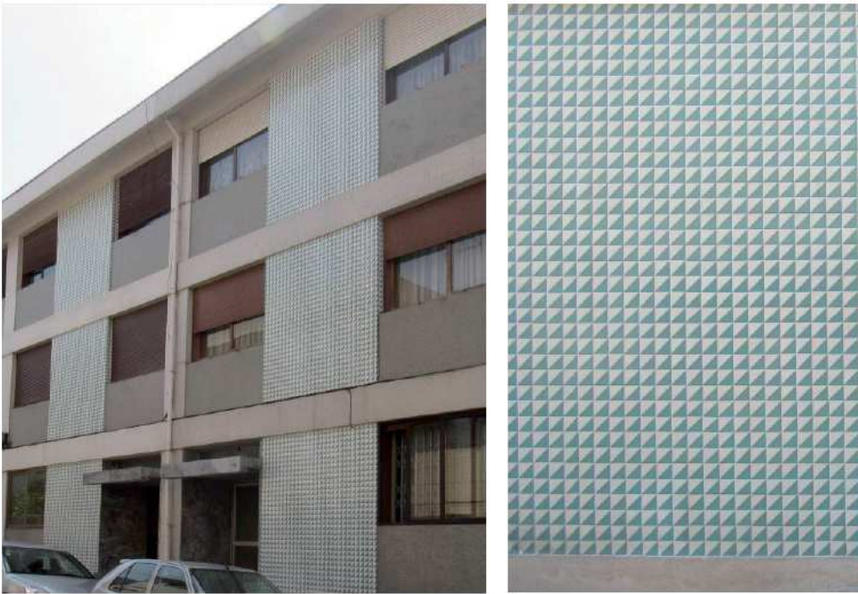
Figure 7: Several buildings in Porto with integrated azulejos. Rua de Bento Júnior N° 97-99
