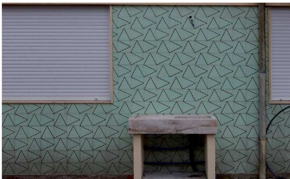
Figure 14: Private house with integrated azulejos in Rua Oliveira Martins Nº 19
