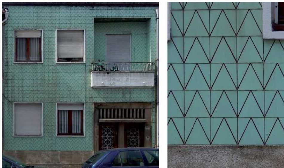
Figure 13: Building with integrated azulejos in Rua Faria Guimarães Nº 257
