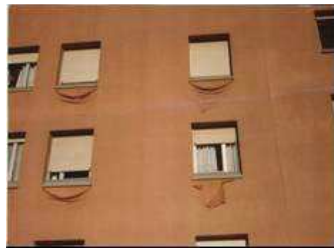
a) Blistering of elastic type painting
