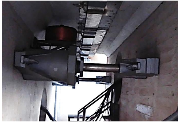
Fig. 4. Anti-seismic device at abutments
