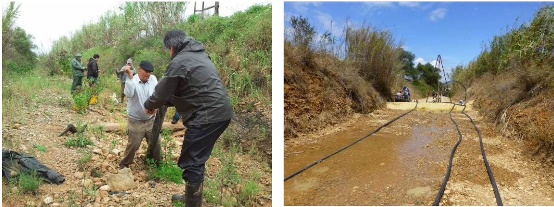
Figure 11 – Rehabilitation of the existing infiltration basins, access and piezometers at PT1_1 Campina de Faro
