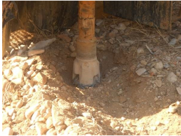
Figure 14 – Rotation with direct circulation
