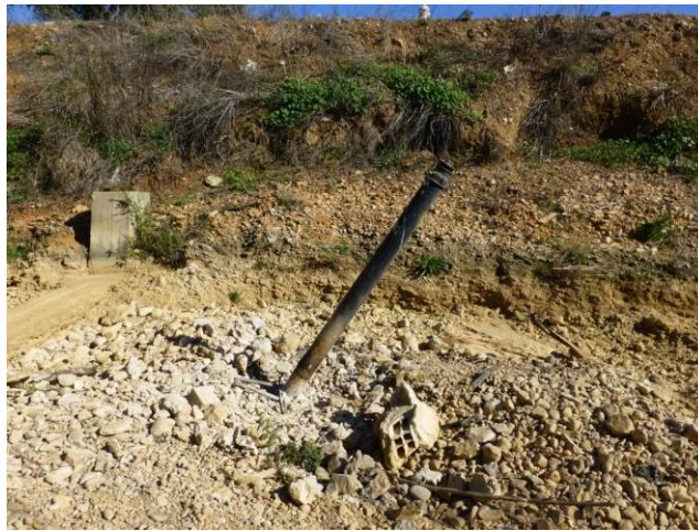
Figure 6 – LNEC1 piezometer before rehabilitation
