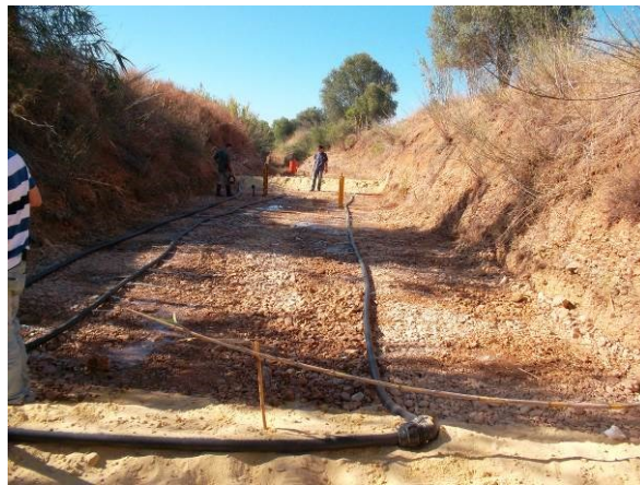
Figure 38 – System of valves to regulate the flow
