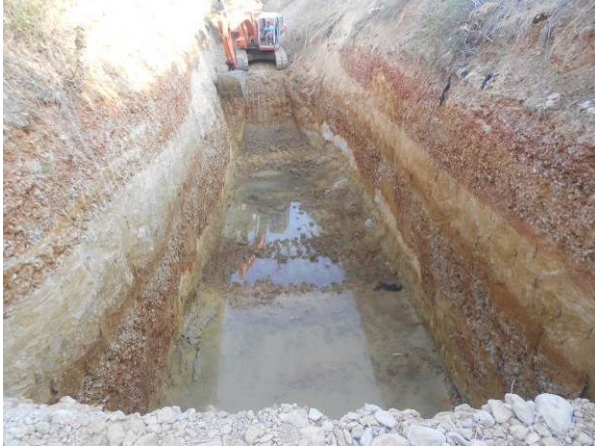
River basin excavation: August 2014
