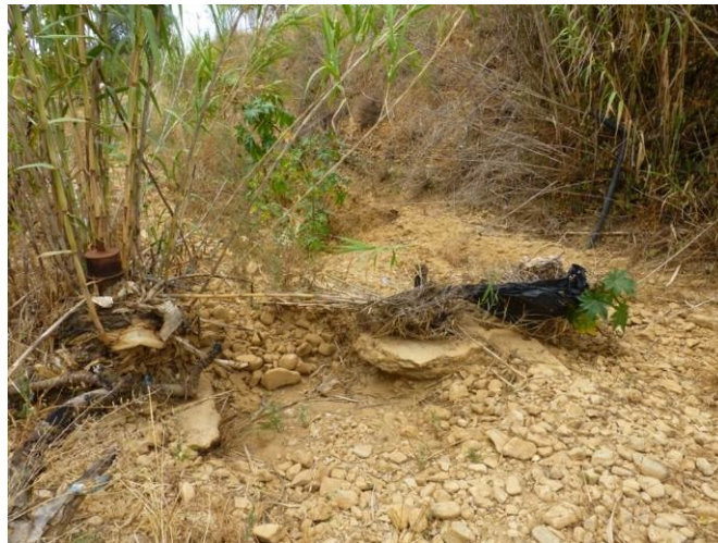
Figure 7 – LNEC2 piezometer and LNEC3 well before rehabilitation
