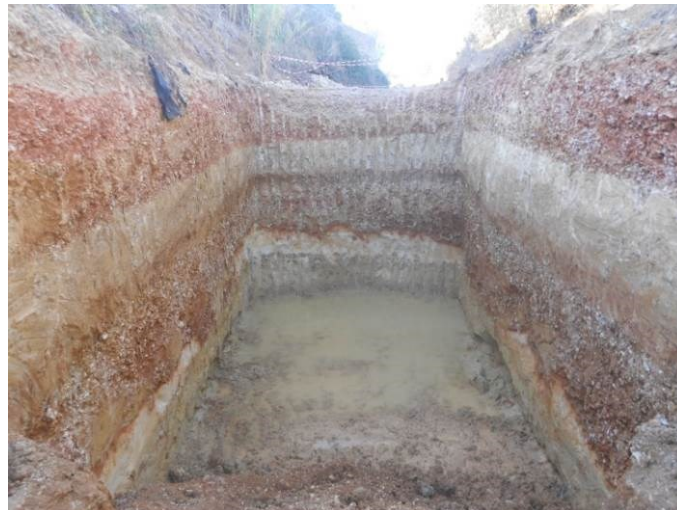
Figure 24 – Lithological levels identified during the excavation of the MARSOL basin
