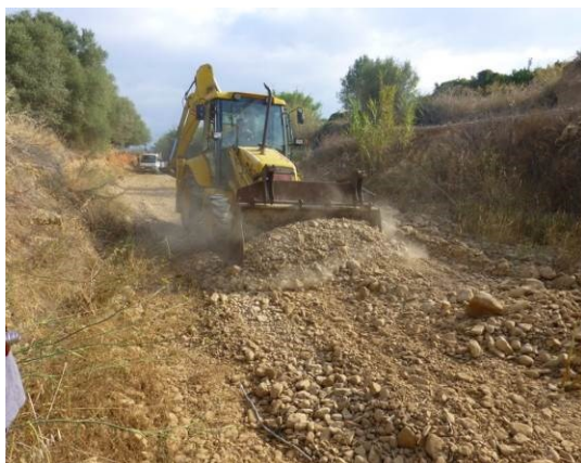
Figure 9 – Levelling of Rio Seco bed
