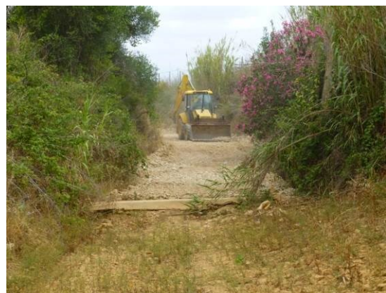
Figure 9 – Levelling of Rio Seco bed
