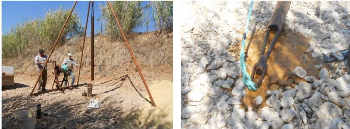
Figure 12 – Piezometer and well development
