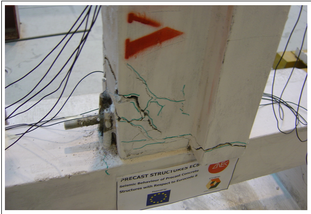
Figure C.39: Specimen VL5 – Detail of the initial cracking.
