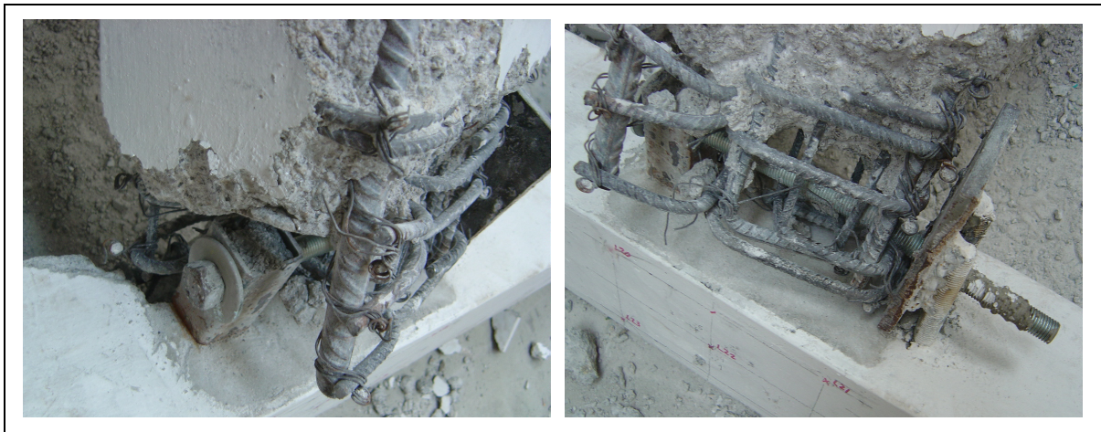
Figure C.32: Specimen VL1 – Reinforcing steel inspection.
