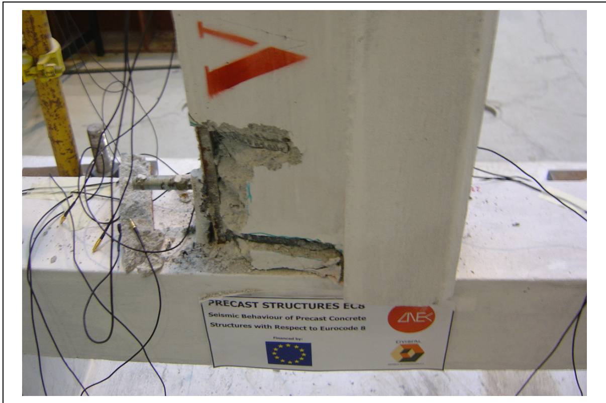
Figure C.37: Specimen VL4 – Detail of the initial damage.
