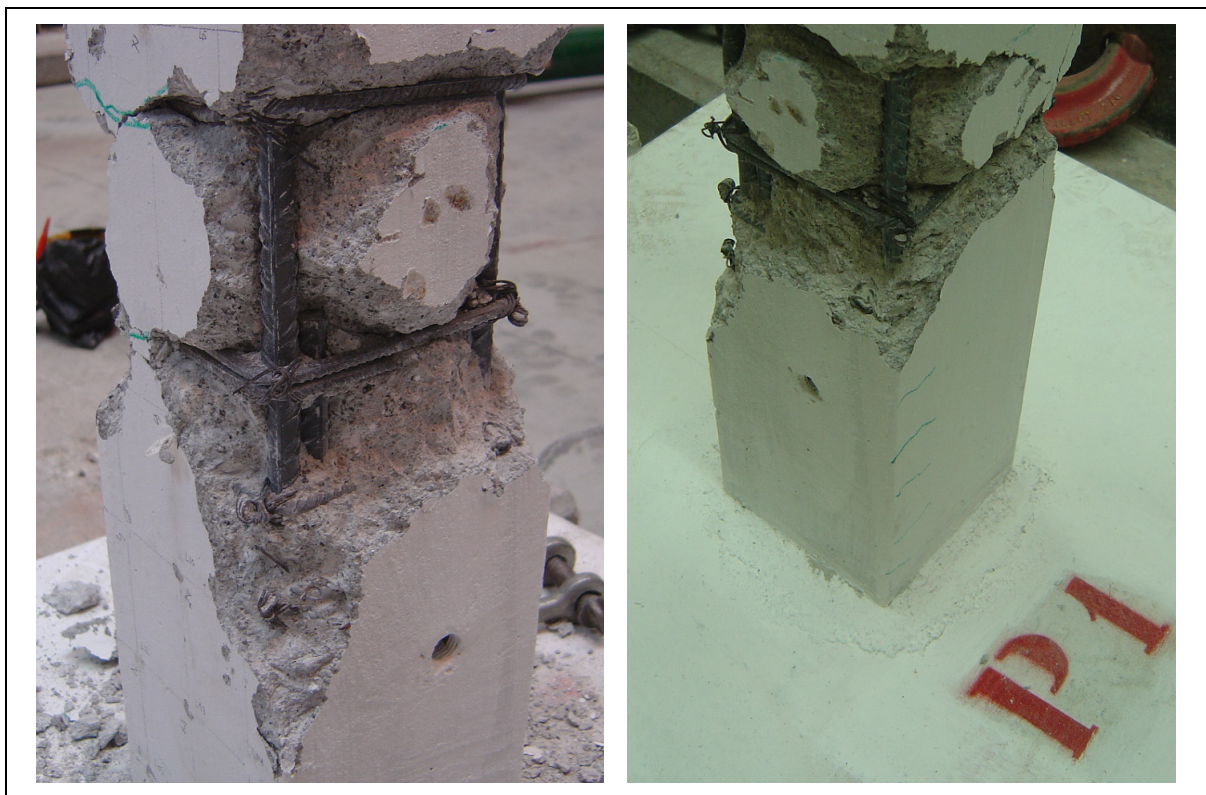
Figure C.6: Specimen P1 – Reinforcing steel inspection and detail of the column-foundation connection.
