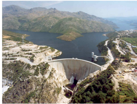
Figure 6: Alto Lindoso dam.
