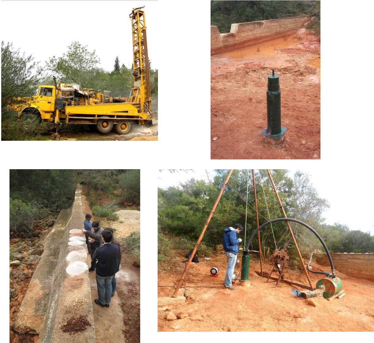
Figure 11 – PT2_6 Construction of two piezometers at Cerro do Bardo DEMO site
