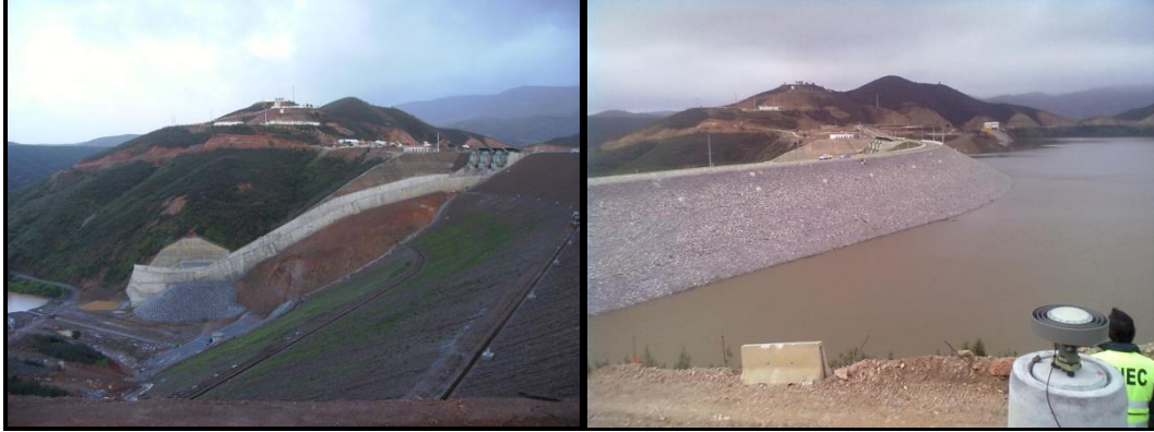
Figure 1: The Odelouca Dam (partial views of downstream and upstream)
