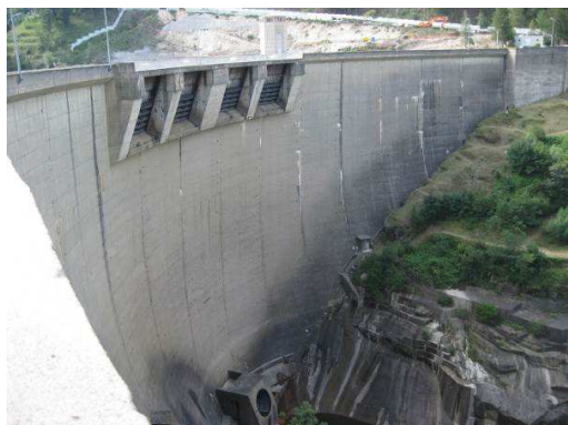
Figure 1: Existing spillway and bottom outlet
