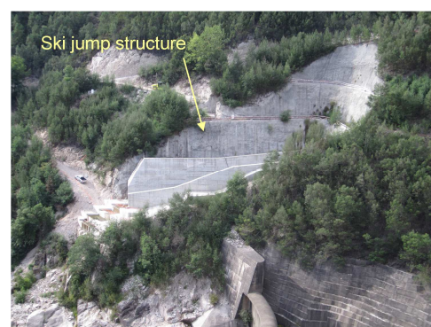
Figure 18: Ski jump structure (August 2014)
