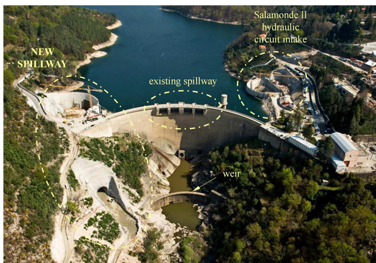
Figure 16: Overview during construction (February 2013)
