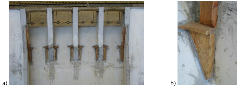
Figure 7: Deflectors in the spillway piers. a) general view; b) detail of the lateral deflector
