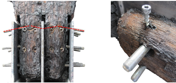
Figure 10: Failure modes of connections D03.1.R-1 (left) and D05.1.R-1 (right) in the fire tests.
