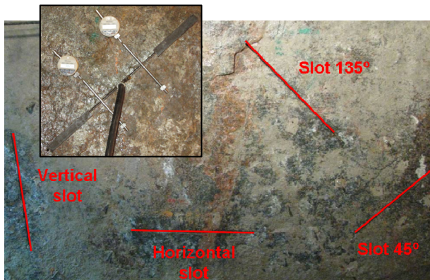
Figure 2. Flat jack array of slots and instrumentation.
