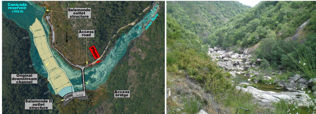
Figure 7. Cávado river nearby and upstream the outlet structure.
