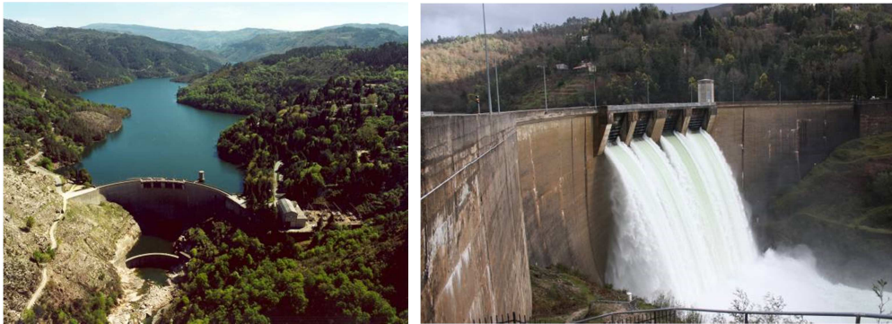
Figure 2. Aerial view of Salamonde dam and spillway in operation.
