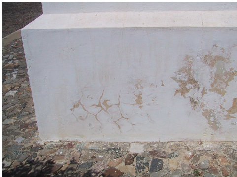
Fig. 18 - Damage seems to start from the cracks (2002-07-03) ... and from other singularities (2003-10-30)
