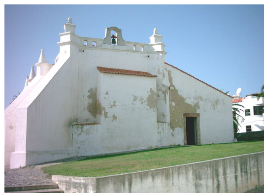
Fig. 6 –Salvas Chapel, NE (back) façade (2003-11-19)
