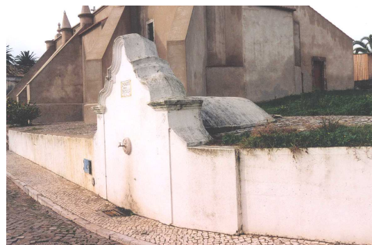
Fig. 4 – Dona Bataça water fountain and reservoir (ancient photo, prior of the most recent interventions) (DGEMN)
