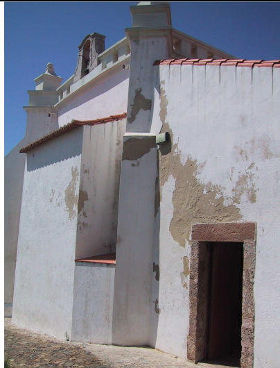
Fig. 10 - NE (back) façade, July 2002
