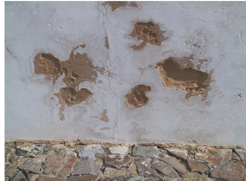
Fig. 18 - Damage seems to start from the cracks (2002-07-03) ... and from other singularities (2003-10-30)
