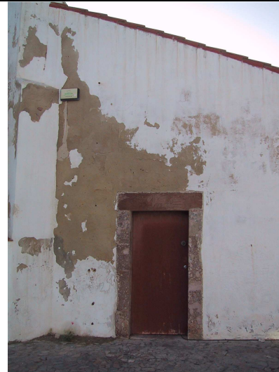
Fig. 11 - NE (back) façade, November 2003
