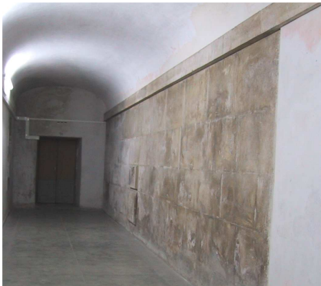
Fig. 11 – Regular stone masonry wall (2004-01-06)
