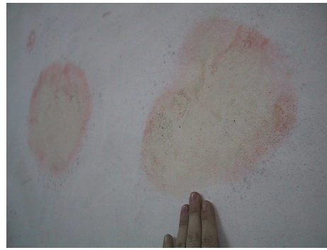
Fig. 16 – Red spots (probably of biological origin) on painted lime-plaster (2004-01-06)
