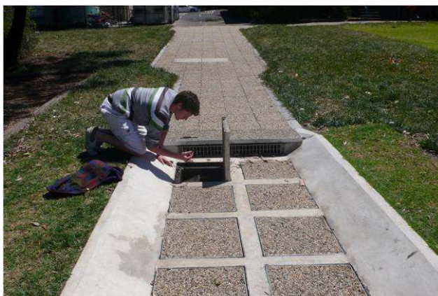
Figure 3-12: Modular filter units for treating storm drainage in Melbourne (can also be associated with street tree pits)
