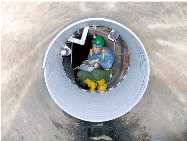
Figure 2-11: Pipe relining (IKT – Institute for Underground Infrastructure)
