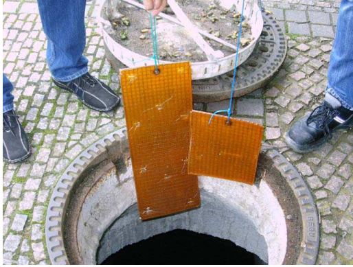
Figure 2-27: Gel-plates before installation in Hannover (Rosenwinkel et al. , 2007)
