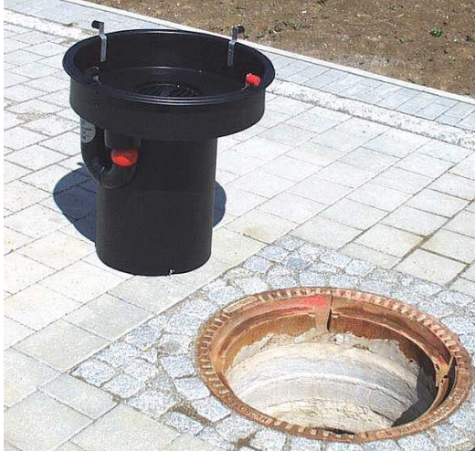
Figure 2-25: Example of a manhole filter (EKO-Biofilter from Warwas)
