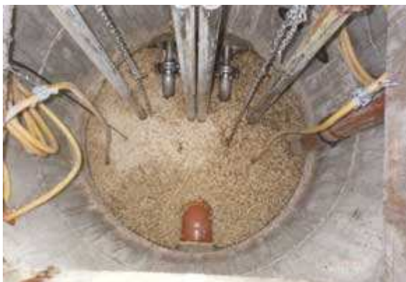
Figure 2-31: Example of amorphous covering system (Unitechnics KG)
