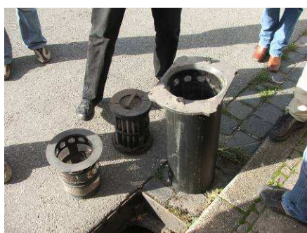
Figure 3-11: the Inolet gully insert filter system to improve runoff quality prior to entry into stormwater sewers (Sommer et al, 2007)
