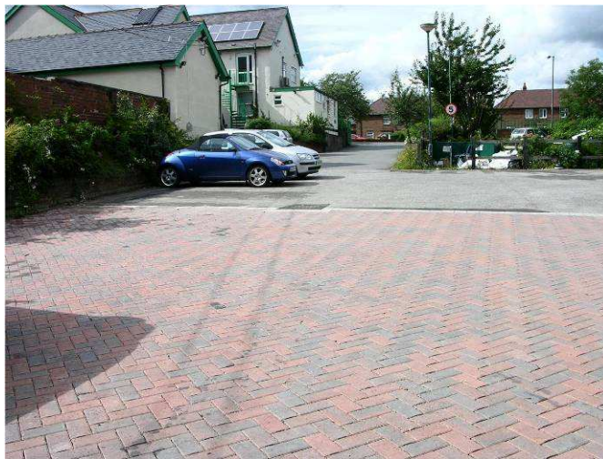
Figure 3-9: Permeable paving at Ground Work Trust - Derbyshire Head Quarters UK that collects the water for heating buildings
